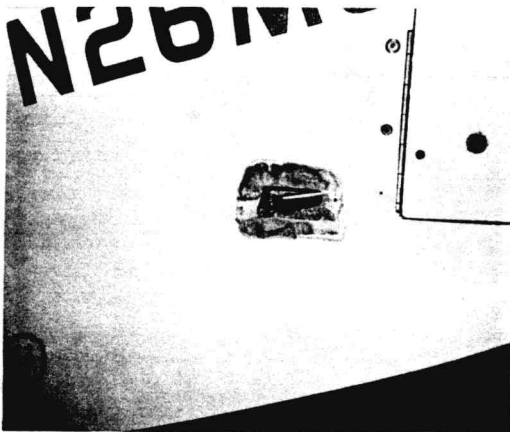
(11) Rudder is temporarily mounted in place and rudder cable end is visible through this access hole in the outboard face of the winglet. Carefully check that rudder travel is sufficient and that there are no hang-ups before covering this access hole with two (2) plies of BID.
